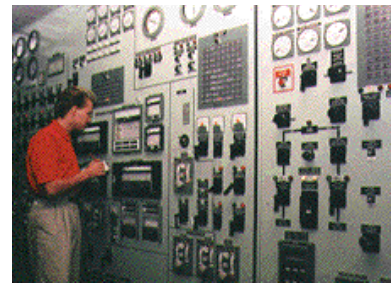
FIGURE 2-3. A nuclear power plant is really just a giant toaster. (Control Room One, D.C. Cook Nuclear Power plant, Ann Arbor, Michigan.)
